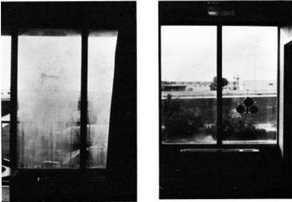
(b) Scummed and Stained Interior Glass Surface
