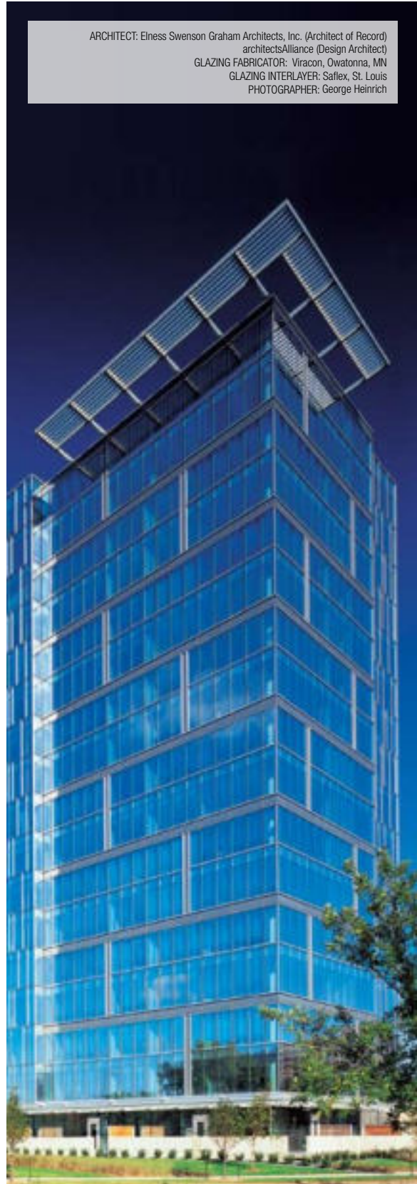
Reflections at Bloomington Central Station: UV & Thermal Glazing featuring Saflex®
